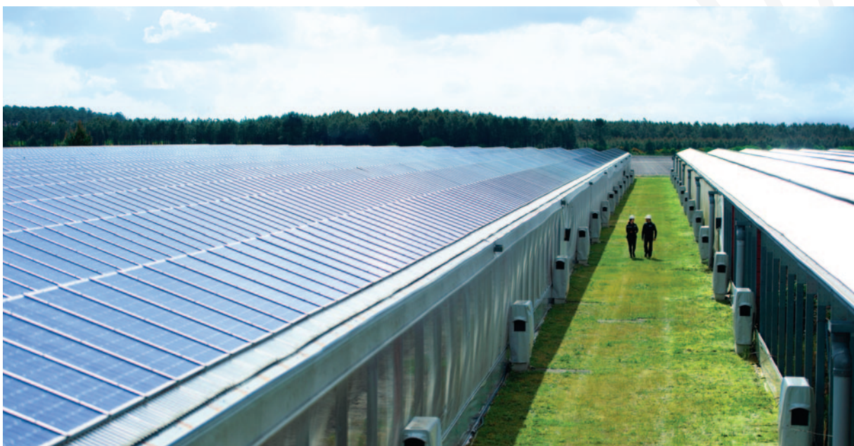
Agri-PV: solar on greenhouses in Lüe, France.
