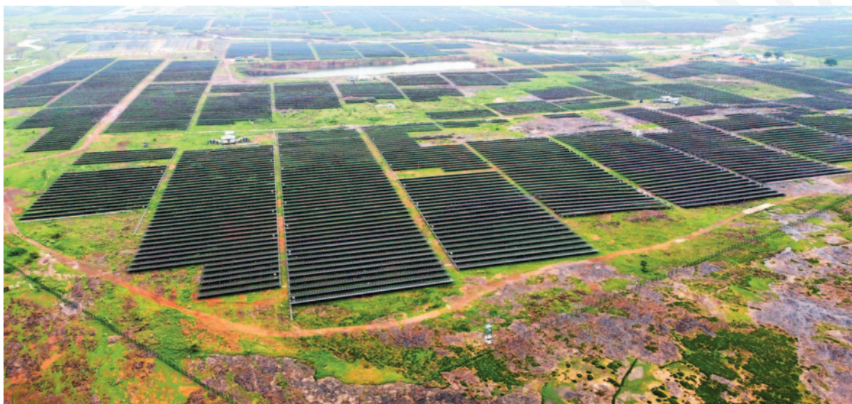
750 MW, Rewa Ultra Mega Solar power plant in Gurh, Rewa, Madhya Pradesh (India).
